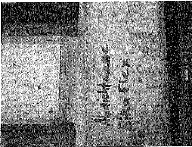
Illustration 9: Transverse bulkhead sealed with sealant mass Sikaflex Tank N (side view and top view)
