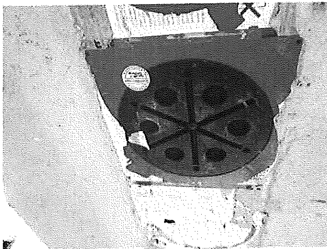
Illustration 22: HSI 150 K2-100 with close-off lid HSI 150-D (1 st experiment), trough under-side after 92 days
